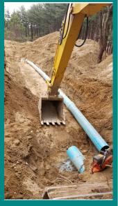
Photo: Installation of underground piping connecting groundwater extraction wells to a PFAS treatment system at BNL.
